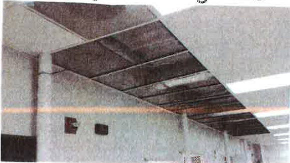
Damaged Ceiling Tiles
